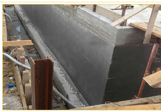
• Waterproofing of concrete or masonry surfaces, under or above ground, such as wells, basins, pools, channels, foundation walls, cellars and elevator pits
